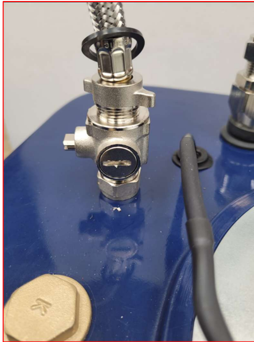
Figure 17: Flow restrictor valve with cartridge inserted and cap fastened securely
